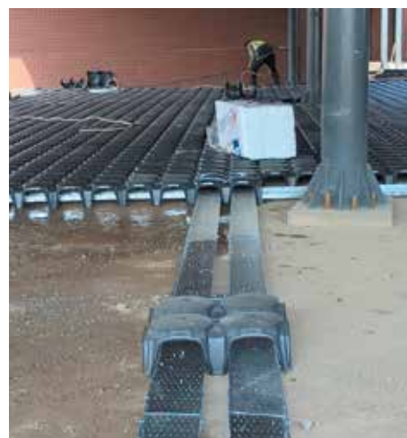
Reinforced Concrete Raised Floor
