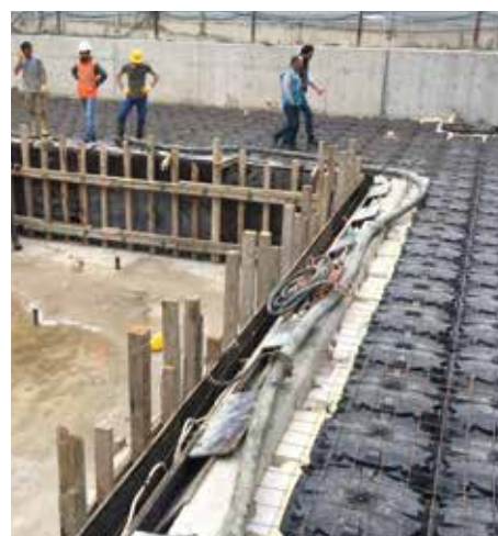
Pool Deck Slab Filling
