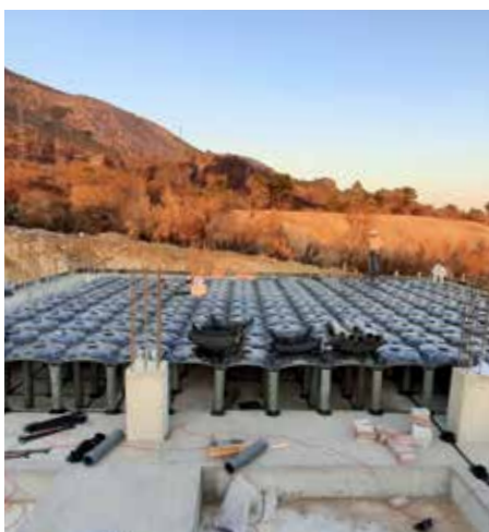
Crawl Space Construction
