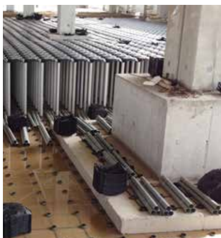
Filling Between Foundation Footings
