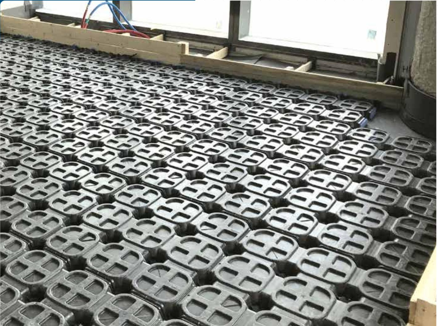
**ABS LEVEL | FIXED-HEIGHT DISPOSABLE FORMWORKS FOR LIGHTWEIGHT FILLINGS (5, 10, 15 cm)**
