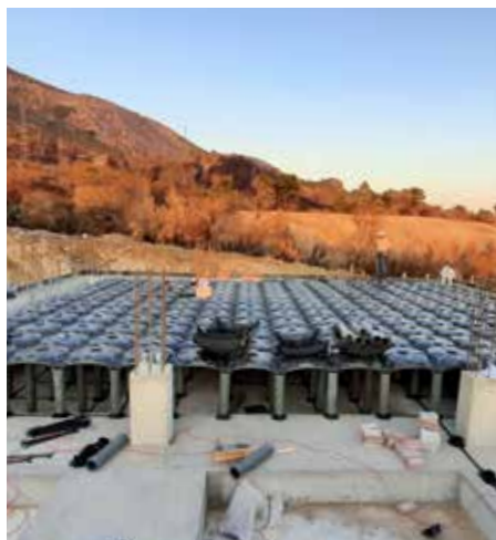
Crawl Space Construction
