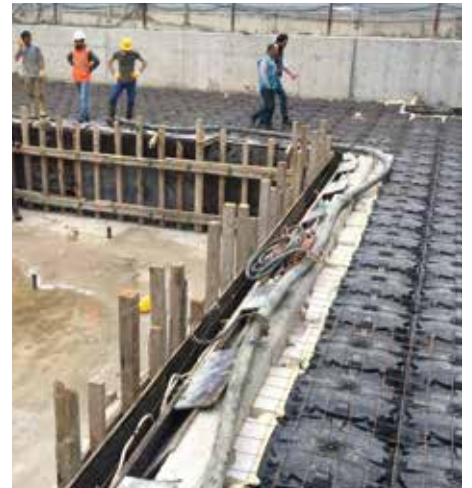
Pool Deck Slab Filling
