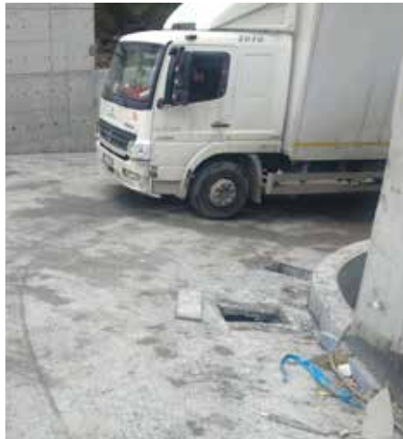
Car Park Ramp
