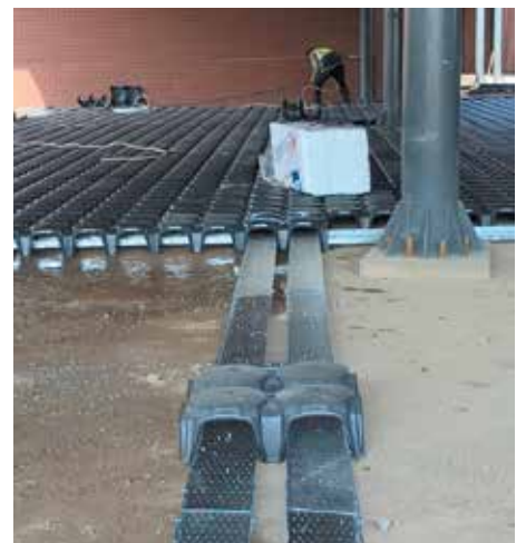
Reinforced Concrete Raised Floor
