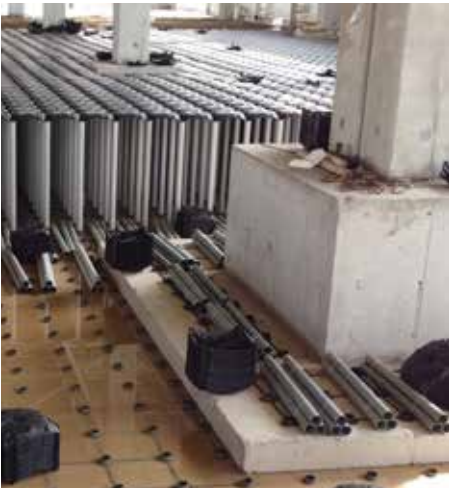
Filling Between Foundation Footings
