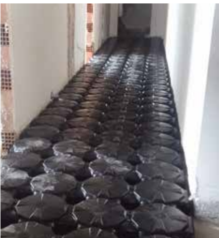
Elevator/Staircase Hallway Filling
