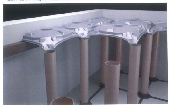
Secure a wooden console on the perimeter wall taking into account the height of the dome to be cut.
