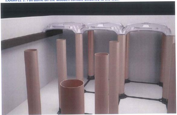
Secure a wooden console to the perimeter wall at the same level as the PVC pipes.
