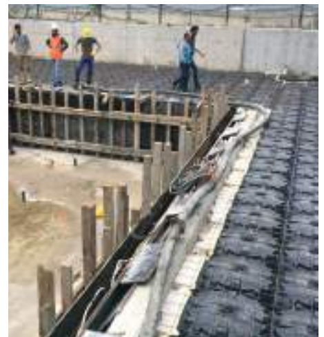
Pool Deck Slab Filling
