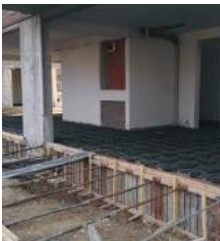
Crawl Space Construction
