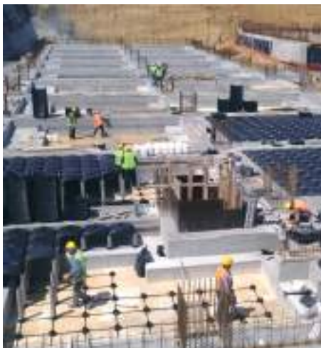
Filling Between Foundation Footings
