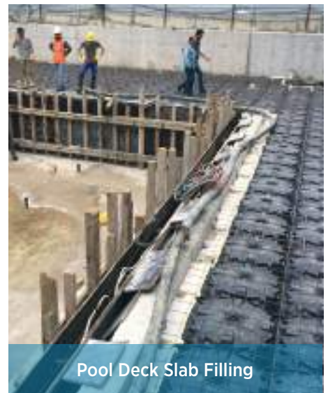
Inverted Beam Filling
