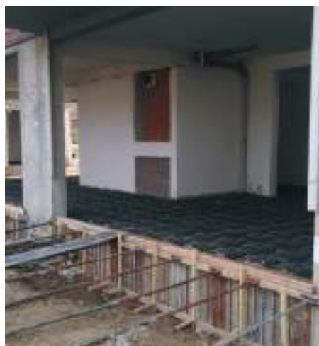
Crawl Space Construction
