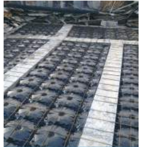
Inverted Beam Filling
