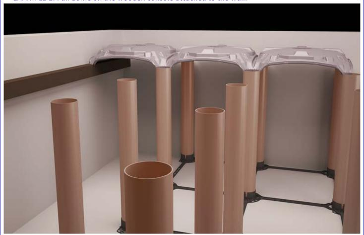
1) Secure a wooden console to the perimeter wall at the same level as the PVC pipes.
