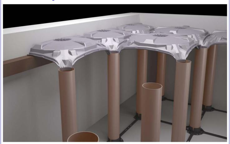
1) Secure a wooden console on the perimeter wall taking into account the height of the dome to be cut.
