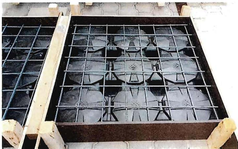
Figure 3: ABS disposable formwork with mesh steel reinforcement prior to concrete casting for sample Group (II) [normal concrete] and Group (III) [fiber concrete].
