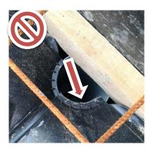
2.4. At the wall finishes, where the PVC pipes stand next to the wall, the space between the dome and the wall must be filled with EPS or wood wedges cut to the appropriate thickness and length. The wedges can be laid upon the PVC pipes freely.
