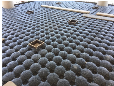
Formworks being laid
